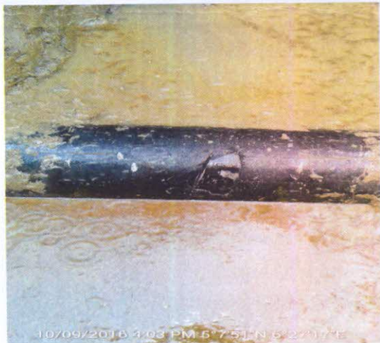
Fig A: picture taken after excavation.
